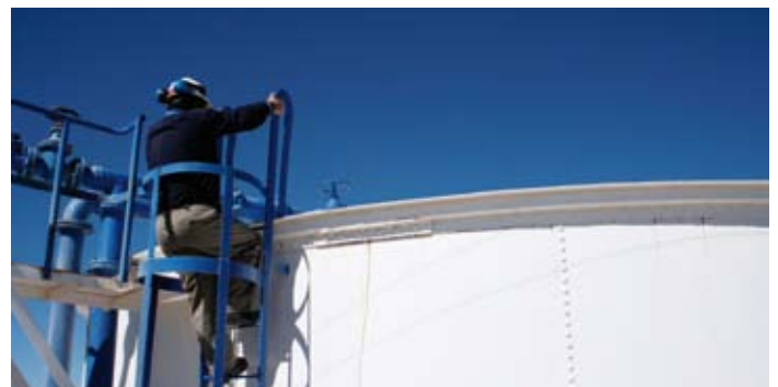
Inspection of water tank
