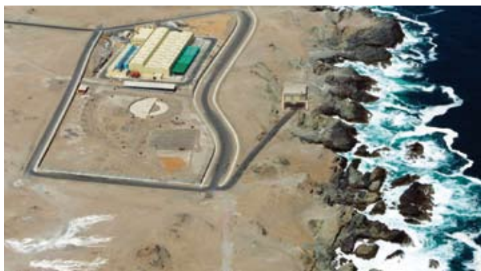
Desalination plant at ADASA
