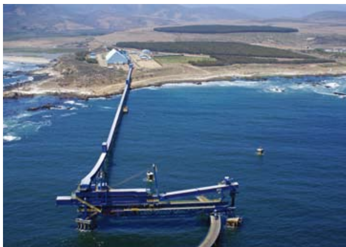
Los Pelambres port facility at Punta Chungo
